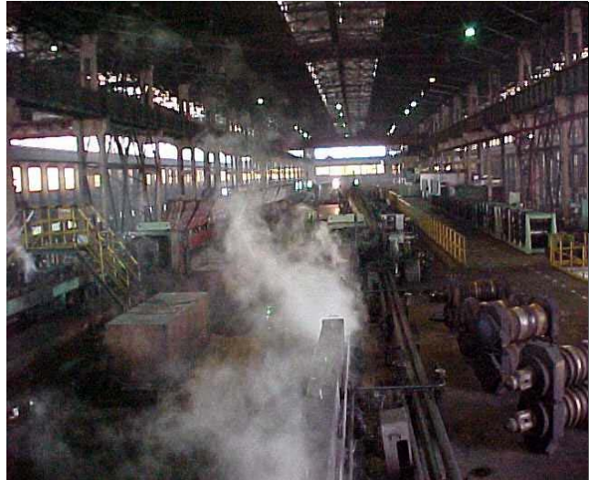
Ma Anshan Steel Wire Rod Mill
