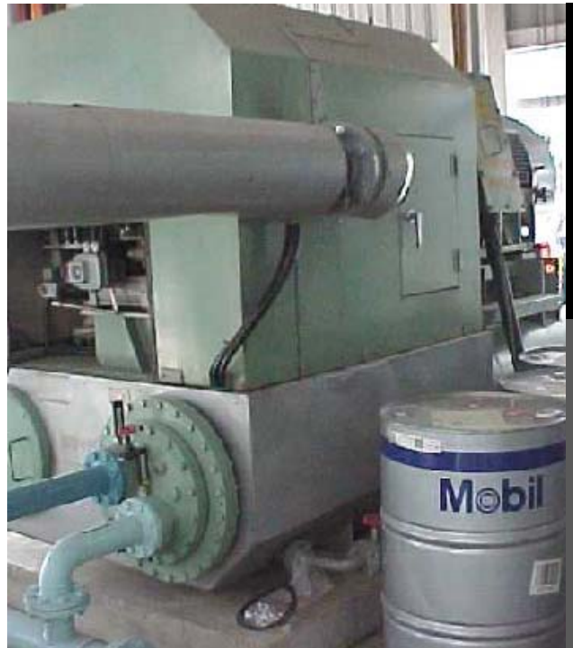
MHI 3-stage Centrifugal Compressor
